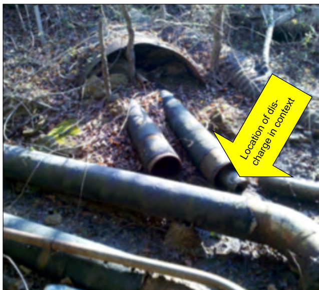
“Big Picture” photo of the pipe and partially filled culvert from which the illicit discharge originates. Provides evidence that can help identify the source of the discharge.
