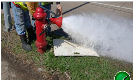
Water Line Flushing
