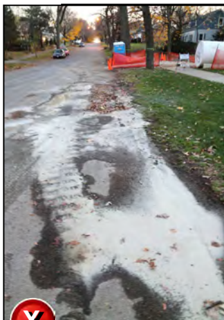
Paint/Plaster/Concrete Washout
