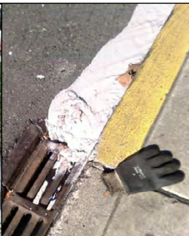
Paint/Plaster/Concrete Washout
