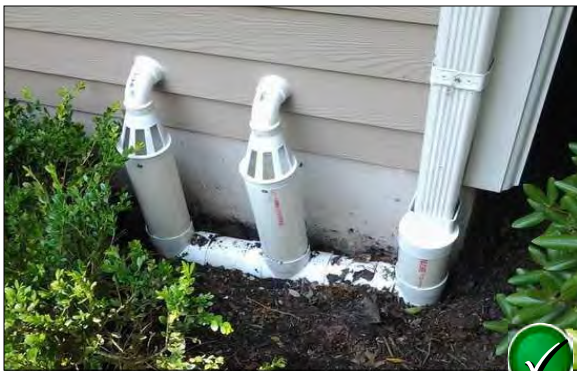
Foundation/Foot Drains & Crawl Space Sump Pumps
